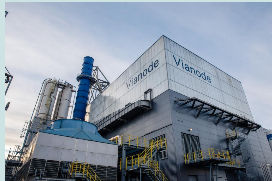
Vianode Via ONE plant
