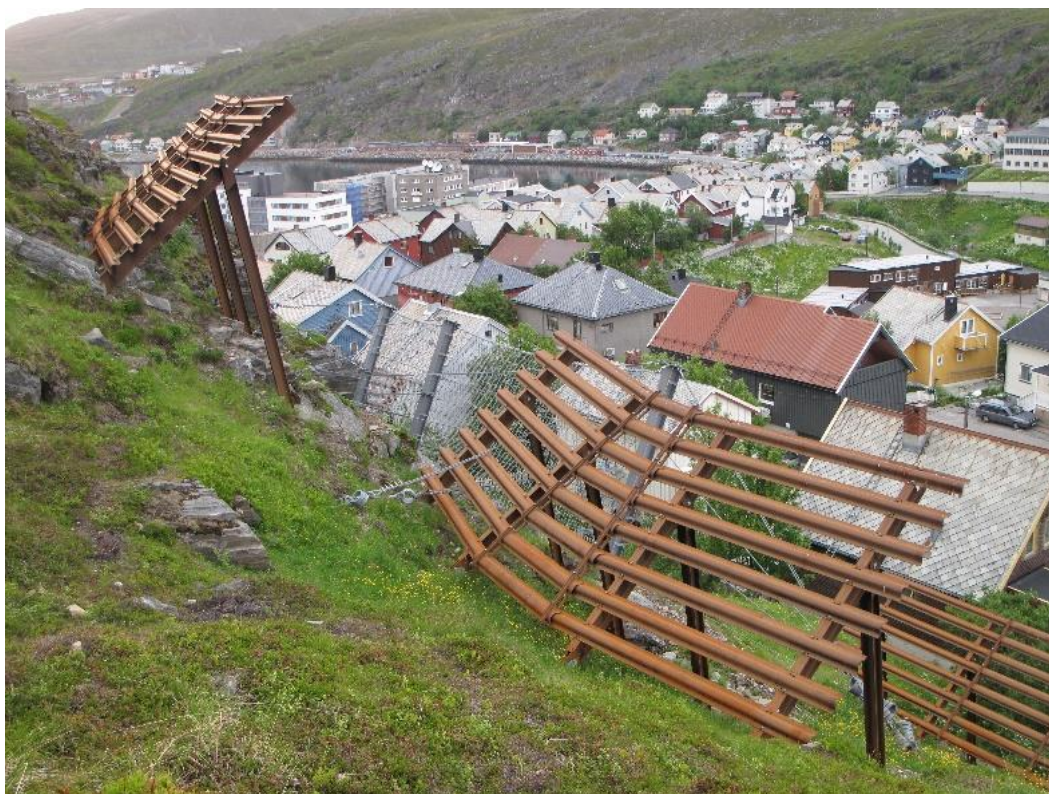
Figure 10. Example of avalanche fens to protect buildings in Hammerfest (Picture: Tom Erik Ness)
